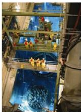
Reactor Vessel Opening / Closing Visual Testing / Surveillance Bolts Replacements
